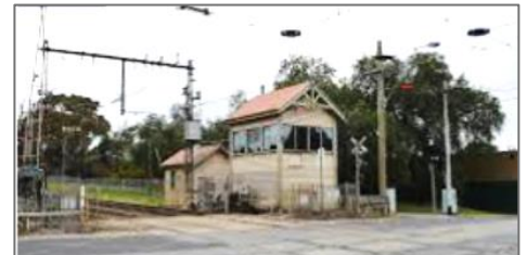
Riversdale Station signal box with its unique boom gates to allow for the trams
