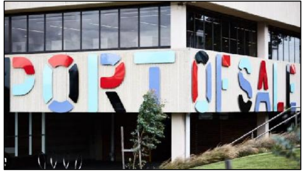
The old Esso building where the Gippsland Art Gallery is now housed.
